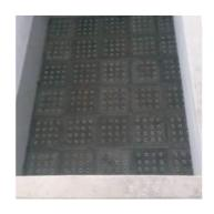
Observation: the plugs are recovered and reused in order to make the next concrete plates.
