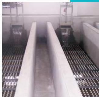
The main component of the nozzles is the filtering element provided with slots of various dimensions (see page 2).
